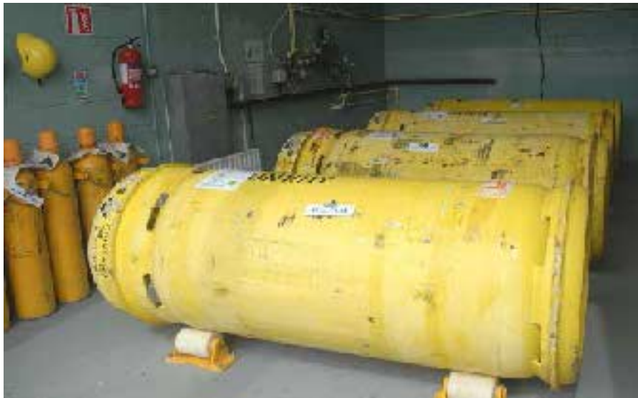
Photograph 3-3: Chlorine gas drums for disinfecting water.
