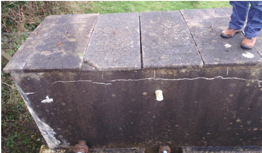
Photograph 3-5: Inadequately sealed clearwater tank/reservoir.
