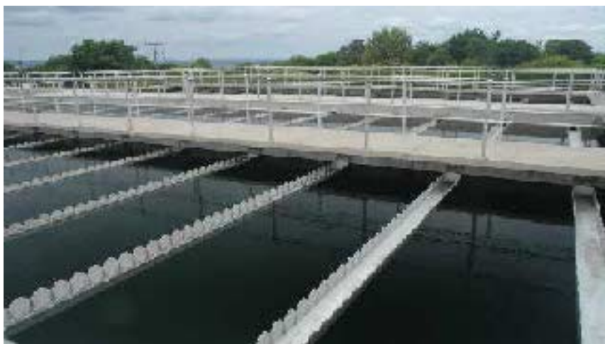
Photograph 3-4: Sedimentation tank.
