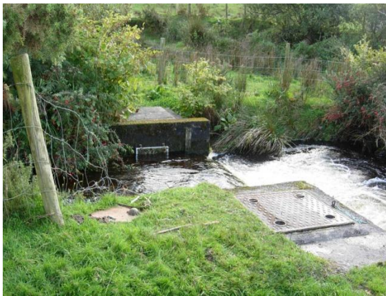
Photograph 3-1: A poorly protected source.
