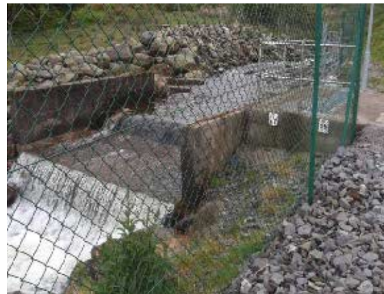
Photograph 3-2: A well protected source with secure fencing around the area of the abstraction point.
