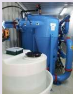
Temporary treatment operating at the Roscommon Central PWS
