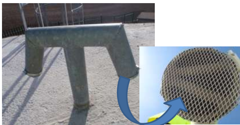
Adequately sealed reservoir vents preventing animal access
