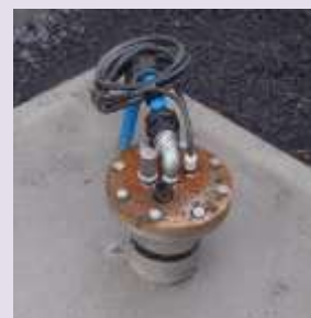
New well constructed at The Strand PWS, Co. Laois.
